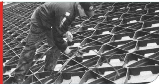
GEORASTER Antierosion Element for Steep Sloped Roofs of 40% - 100% of Pitch
